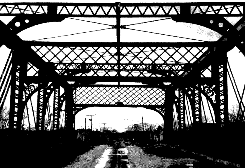
Above: The Selby Avenue Bridge, panorama, detail, and the strip of names cast on retaining and abutment walls.
