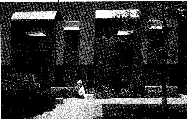
Below, opposite page: Daybreak Grove Photos and graphic: René Davids, Christine Killory
