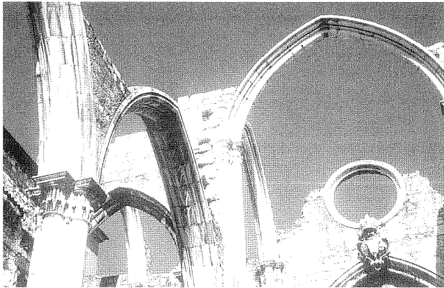
Ruined Gothic vaults of the Cathedral of Carmo, destroyed in the 1755 earthquake and left as a monument.
