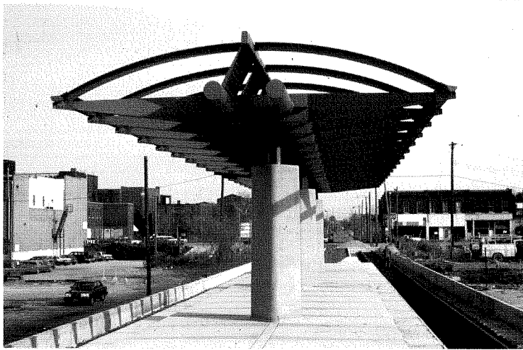
Left: East St. Louis Station canopy structure before sheathing. Courtesy Alice Adams. Above: Historic architectural remnants incorporated into design of Delmar station at the recommendation of the artist team. Courtesy Alice Adams.
