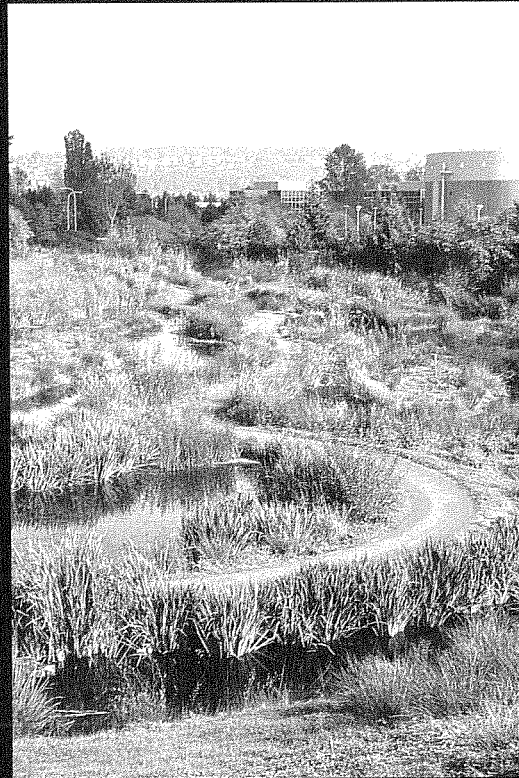
left: The Release, the fifth and final garden room, where cleansed water flows from the last stormwater treatment pond to the enhanced wetland and then to Springbrook Creek.
